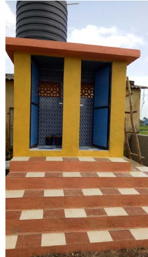
Modular Toilet at Mundhewadi Zila Parishad School, Asangaon
